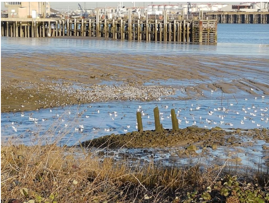
Photograph 2: Sewage outfall channel in Compartment 3 – note flocks in water and on adjacent banks
