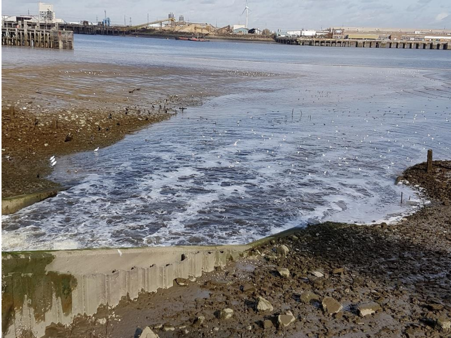
Photograph 1: Sewage outfall channel in Compartment 3 close to low tide
